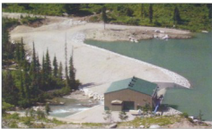
Completed Intake Structure on Pingston Creek
