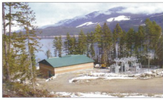
Powerhouse Located on the West Shore of Upper Arrow Lake
