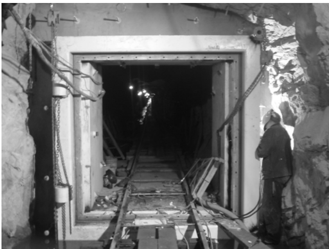
Figure 8. Upper Tunnel Plug – upstream end showing door hinge on left.
