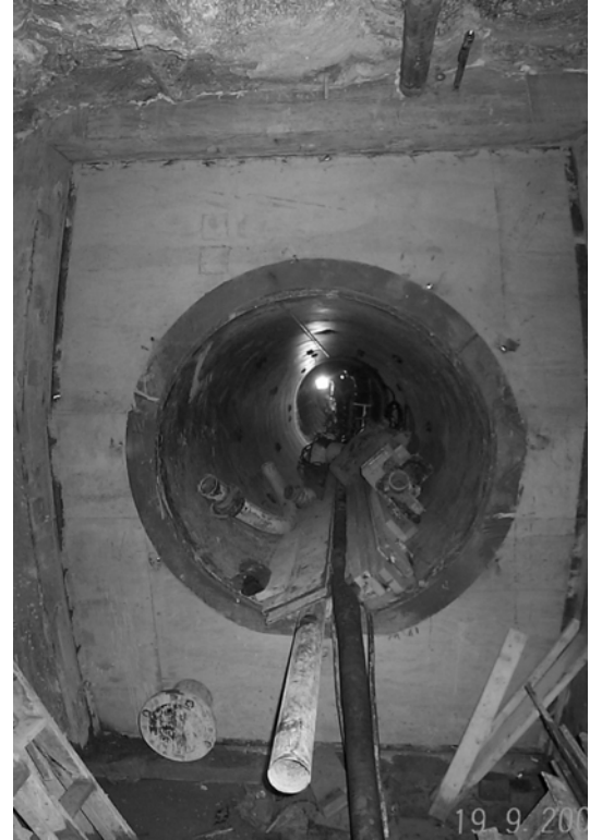
Figure 7. Lower Tunnel Plug – upstream end.
