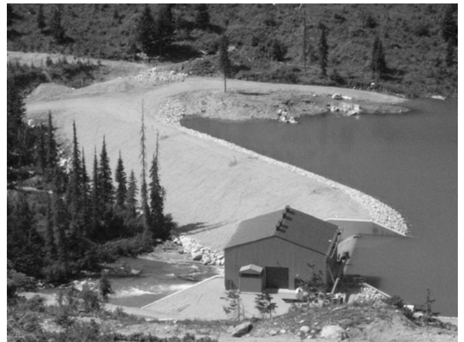
Figure 4. Intake structure and headpond
