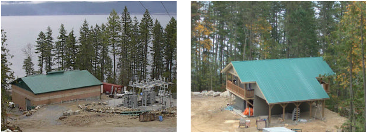
Figure 4: Pingston Powerhouse (left) and nearby Maintenance Building (right).
