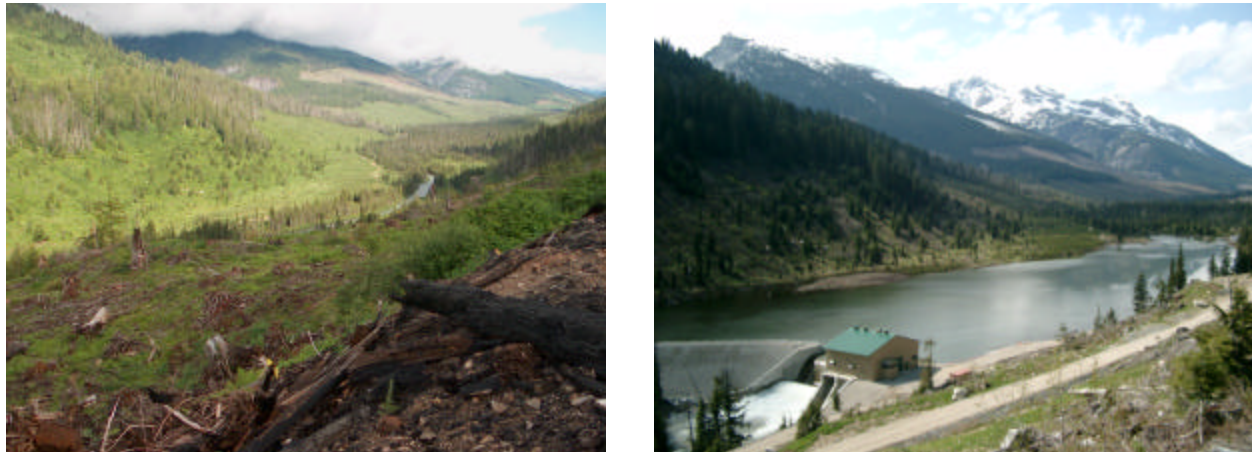
Figure 2: Pingston Creek headworks area and watershed during initial site investigations (2001) and during the 30 MW plant commissioning (2003).
